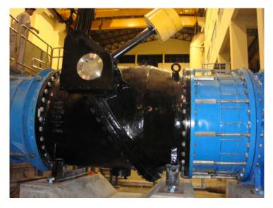
The tilting disc check valve shall consist of a circular disc with conical rim, hinged about a fixed pivot above its center-line and offset from the plane of the seat, sealing against a body seat clamped between the two sections of the valve body.
